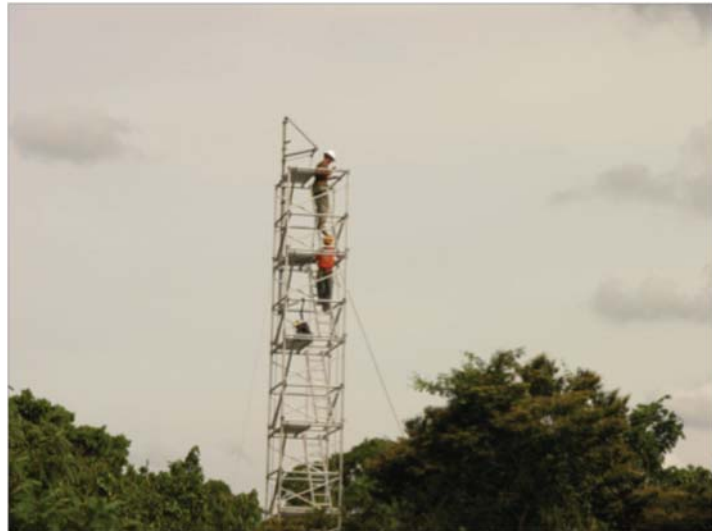
Figure 1. Construction of one of the aluminum walk-up towers at La Selva.
