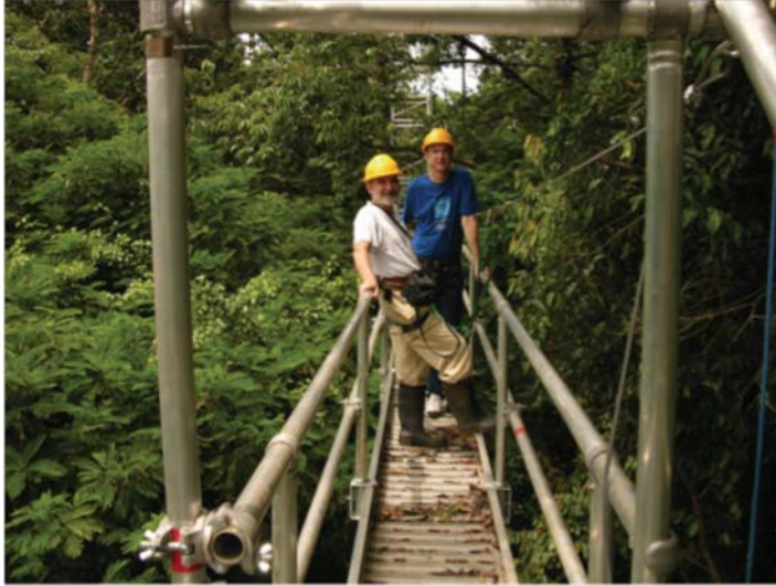
Figure 2. The canopy walkway extends for 25 m, connecting two of the walk-up towers, and is positioned 25 m above ground at the height of the crowns of the emergent trees.
